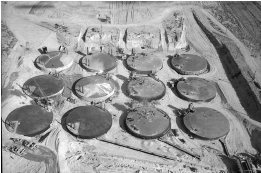
A tank farm at Hanford
